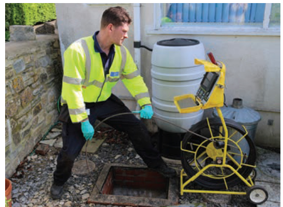
Carrying out a CCTV survey
